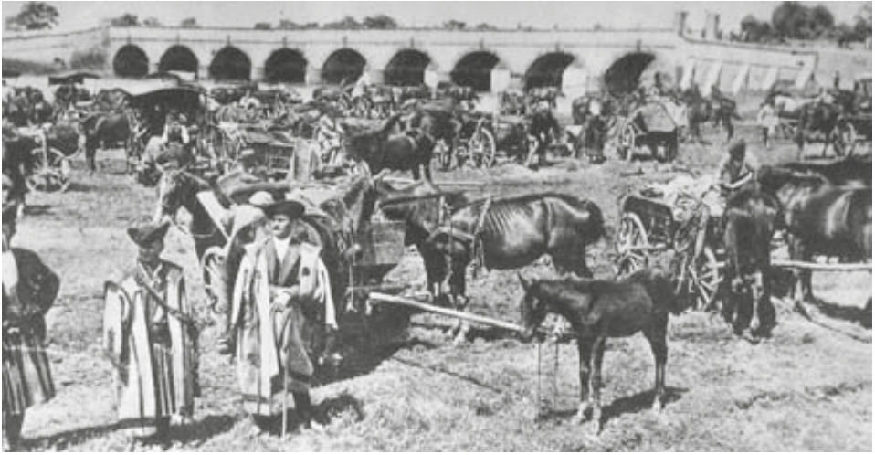
Fig. 1. The bridge fair in 1930
